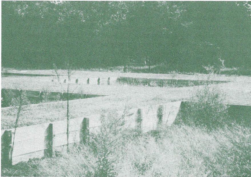
Figure 2. Construction detail of ponds with vertical sides, using wooden boards to minimize leakage and erosion
