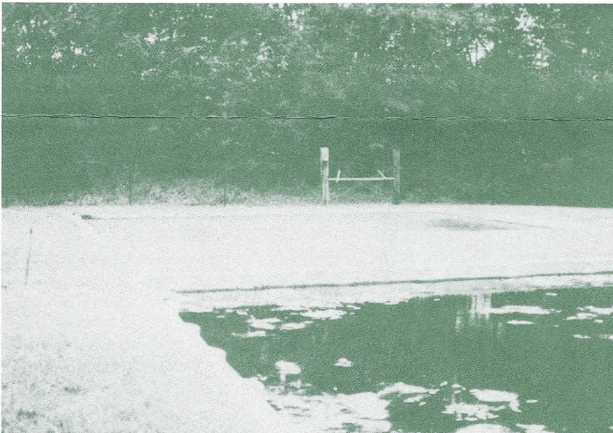
Figure 3. Ponds with wooden sides after application of sprayable concrete to further minimize leakage
